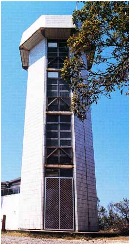
The unmanned Fitzroy Island Lighthouse near Cairns in Queensland, built of tiled concrete in 1973, replaces the original manned light built in 1943.
