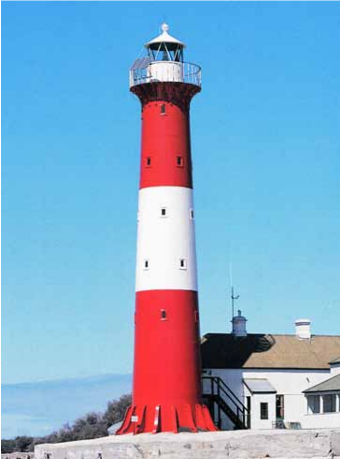
Troubridge Island Lighthouse in St. Vincent's Gulf, was the second lighthouse to be built in South Australia, in 1856. It was the first to be built of cylindrical cast iron segments imported from England and assembled on site.
