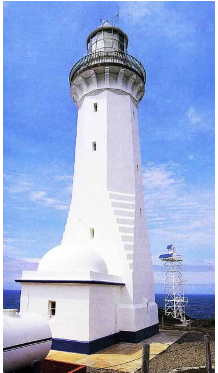
Green Cape Lighthouse in southern NSW was designed by government architect James Barnet, and built in 1883, was the first concrete lighthouse in Australia. It is no longer in use, replaced in 1998 by a steel lattice tower close by.
