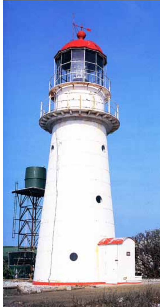
Booby Island Lighthouse, on an island in Torres Strait off the Queensland coast, was built in 1890. It is one of several Queensland lighthouses to be built with a timber frame and galvanised iron panels.
