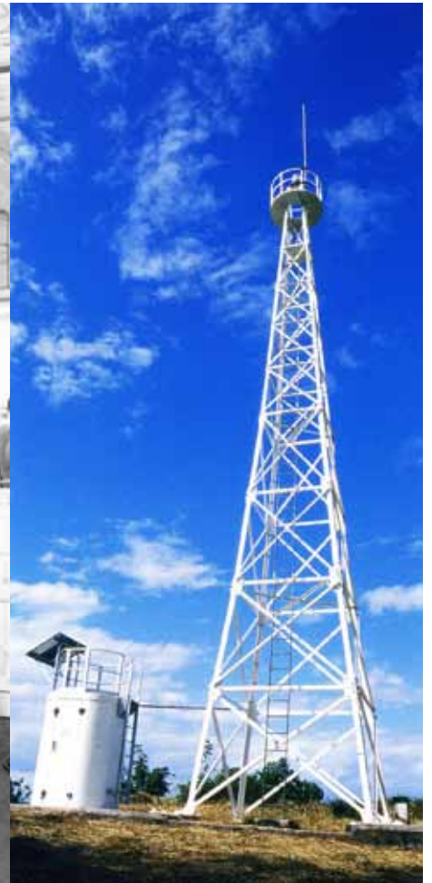
South Brook Island Lighthouse is a steel framed structure off the Queensland coast near Cairns. It was built in 1921 and there are several others like it.
