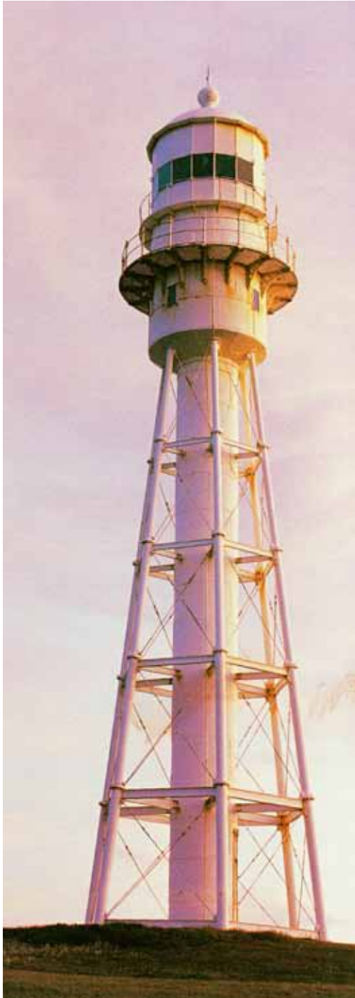
Currie Harbour Lighthouse, on King Island, built in 1880, was prefabricated from cast iron and wrought iron sections in Britain and assembled on site. The light was extinguished in 1989 but relit in 1995 following a public protest.
