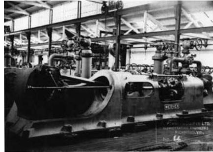
100 ton compressor in erecting shop, 1912
