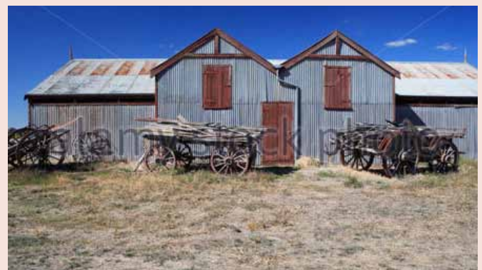
Corrugated iron building at Rutherglen,
