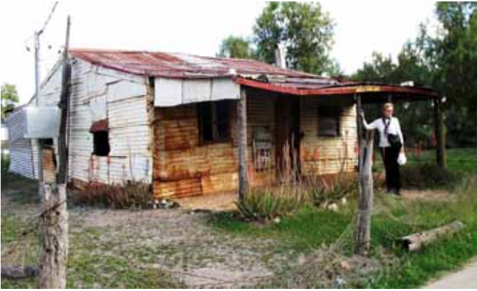
Opal miner's cottage at Lightning Ridge
