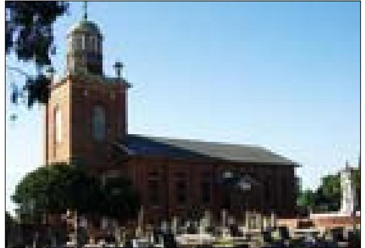
St. Matthew's, Windsor designed by Francis Greenway
