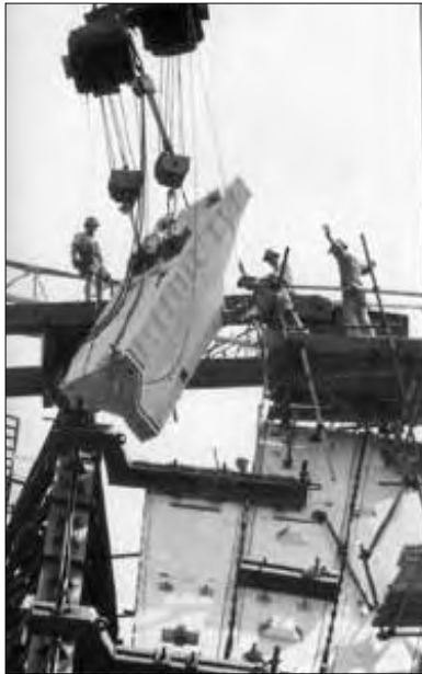
Lifting a rib section
